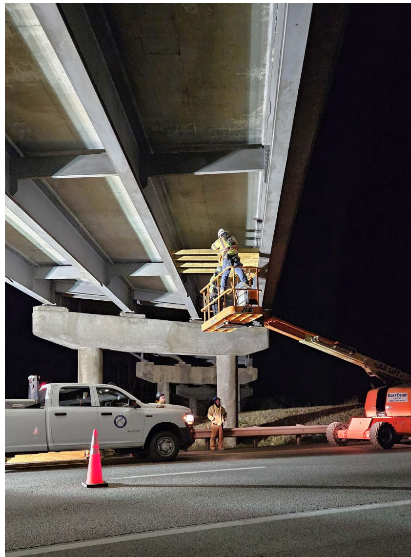
Contractors preparing for removal of existing Route 635 bridge over I-81
